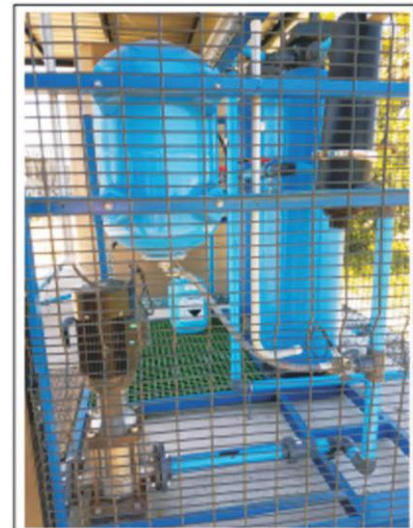
SKID SET UP.
